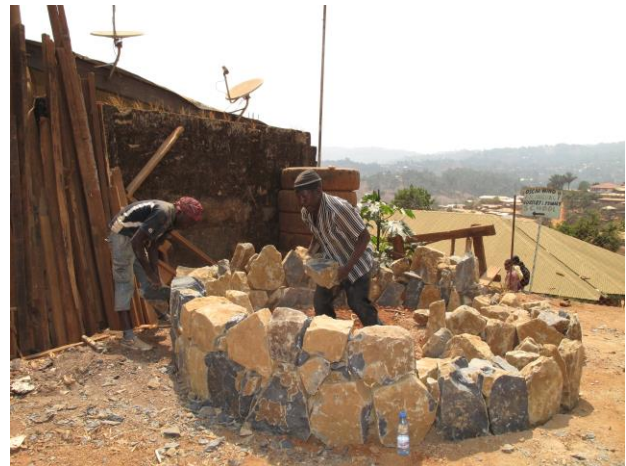
Above: Construction begins at Oscar Wind School.
