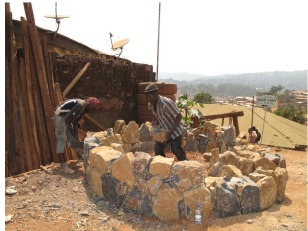
Above: Construction begins at Oscar Wind School.
